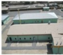
Figure 2 - Southern Portion of Imam Sahib Border Police Company Headquarters
