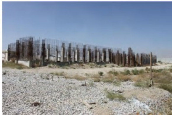
The incomplete courthouse at Parwan.
