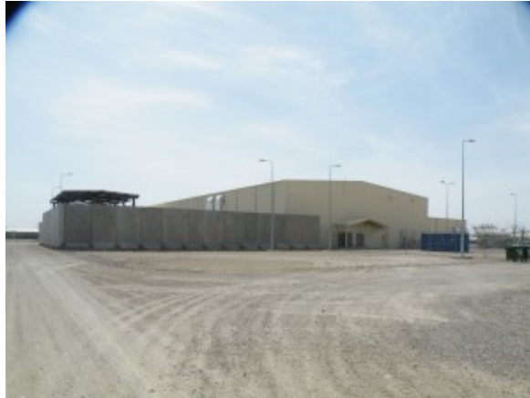
The $34 million building without a use. (SIGAR photo)
