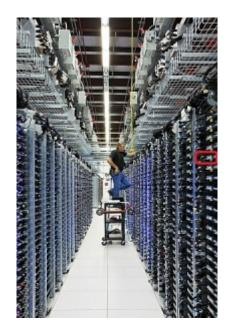
Beneath those white tiles making up the 'floor' are miles and miles of network cables and wiring for power as well as ventilation systems. More cables, wires, and ventilation run overhead.
